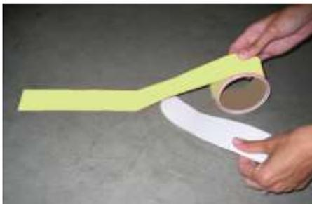
Firmly rub or roll the tape in the same direction as it was applied on the initial pass. Repeat rubbing or rolling as necessary to insure tape has completely conformed to the surface. Premium construction adhesive can be applied to the tape or installation surface as necessary to improve adhesion to slightly rough surfaces.
