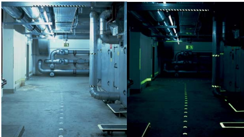
Utility Bunker with obstacles and exit path marked.
